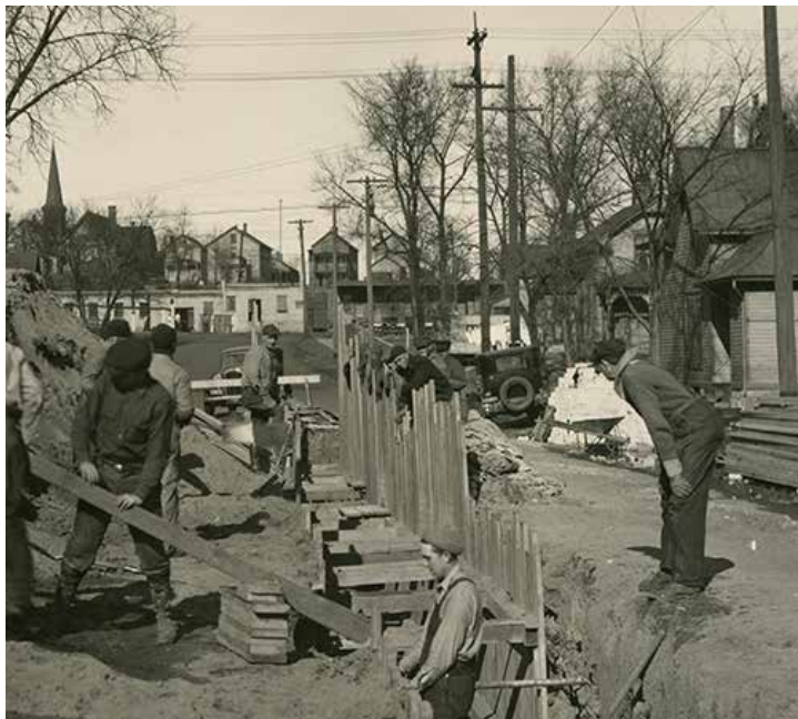
Civil Works Administration workers in Minnesota repair a sewer. Credit: FDR Presidential Library and Museum
